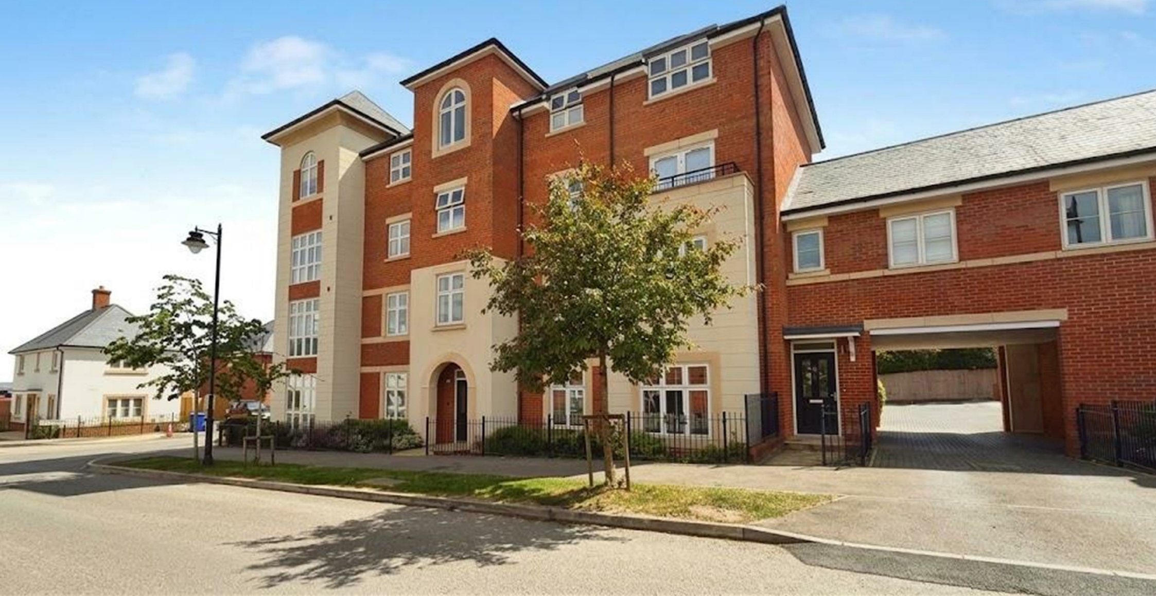
10 Islander House Montgomery Avenue, Wellesley
