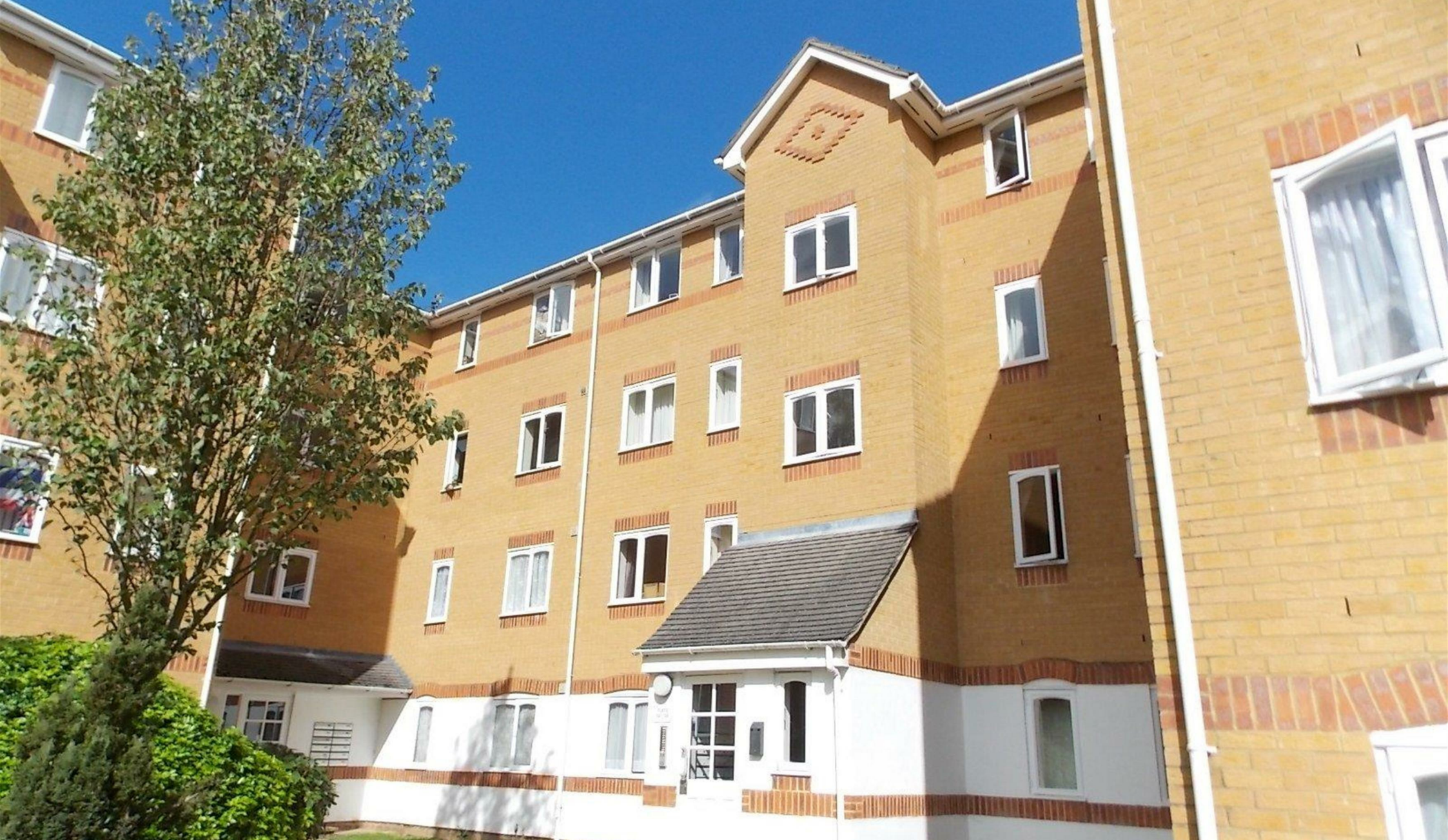
Ascot Court, Grove Road, Aldershot
