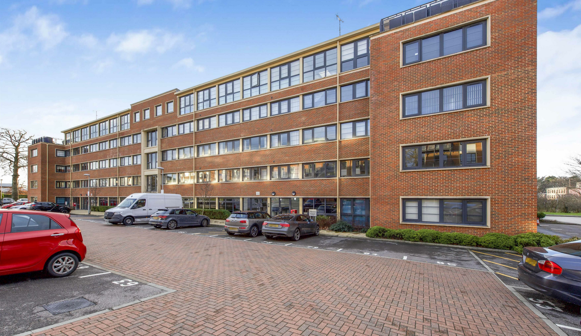
Wessex Court, Kestrel Road, Farnborough
