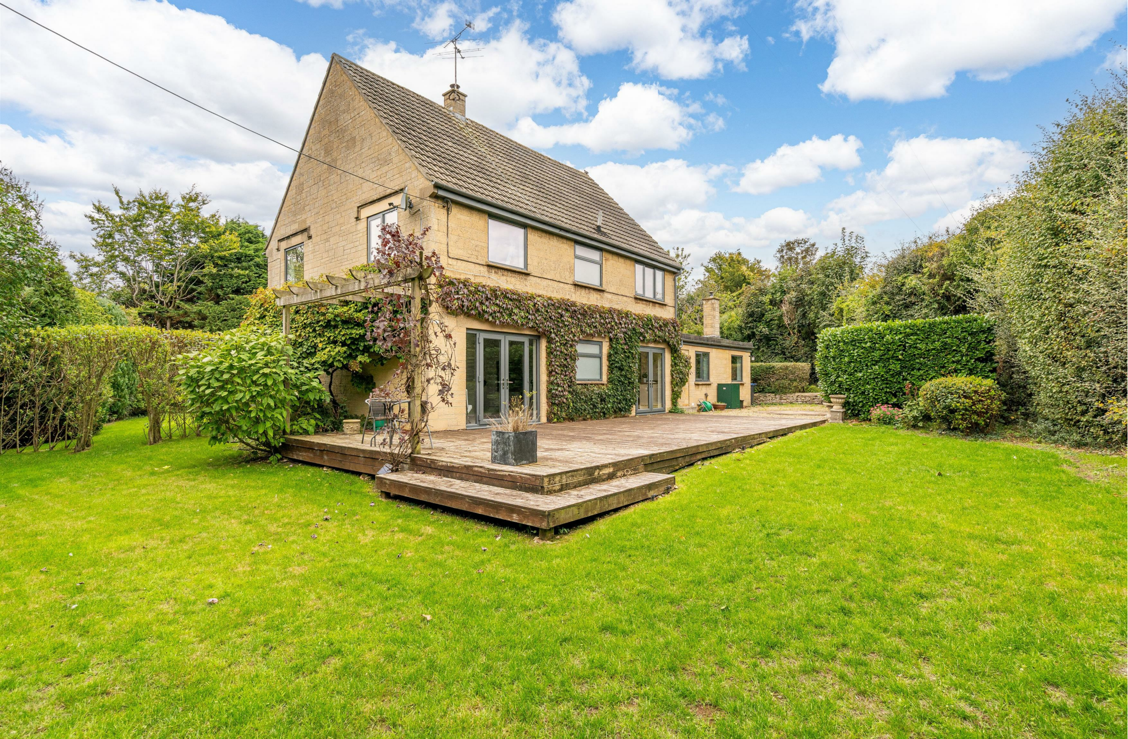
Showing the rear garden and decking with access from the living room and kitchen patio doors
